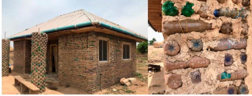
Şekil 2.4. Bottle house in Païpe, Abuja, Nigeria.
